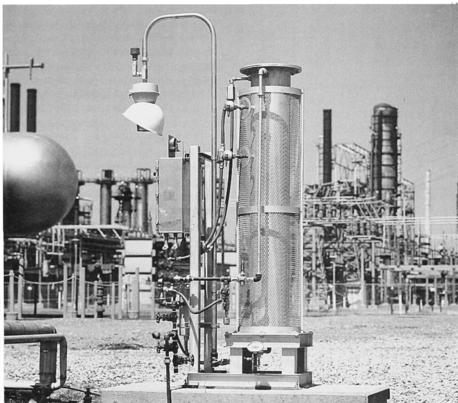
The Thermatrix system, which destroys hazardous air pollutants, was developed by the Department of Energy and commercialized by a private U.S. firm.
