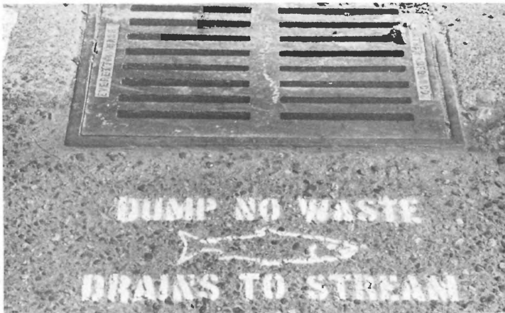
"Adopt-a-Stream" groups are painting storm drains, such as these in Bothell, Washington, with this explicit warning. The goal is to restore polluted water bodies such as Puget Sound.
