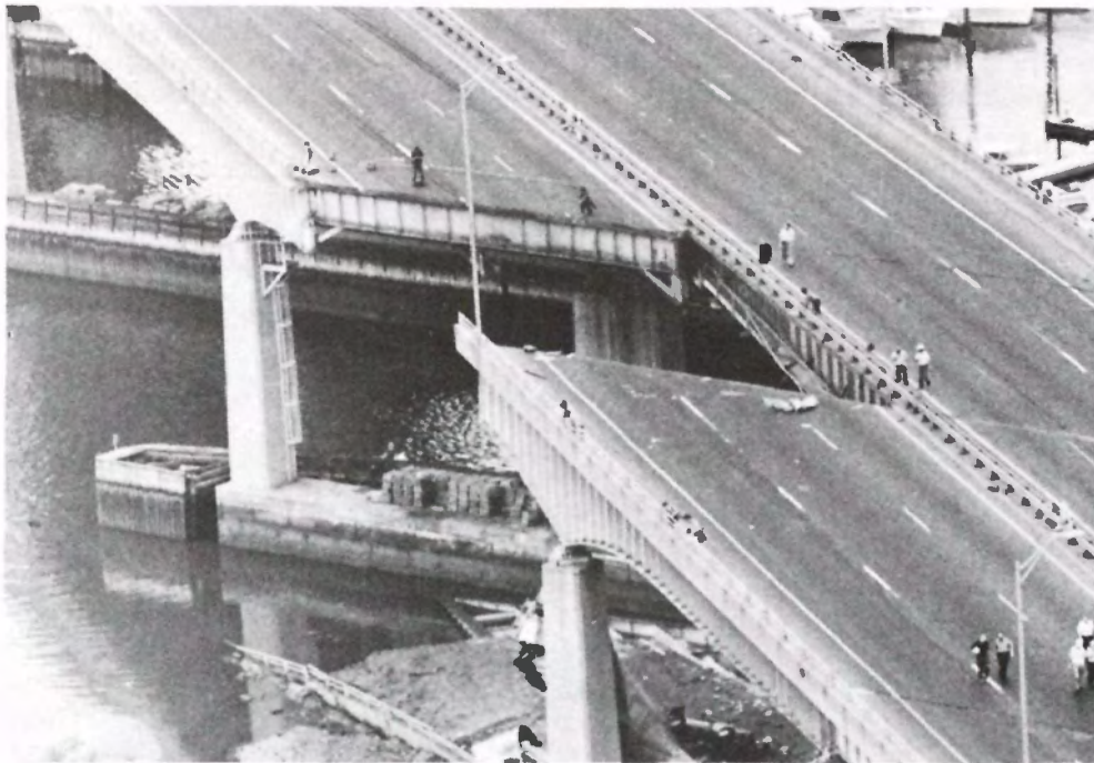
The collapse of a 100-foot section of Connecticut Turnpike Bridge into the Mianus River in June 1983 caused many states to intensify inspections of pin-connected bridges. Sara Krulwich photo, New York Times Pictures.
