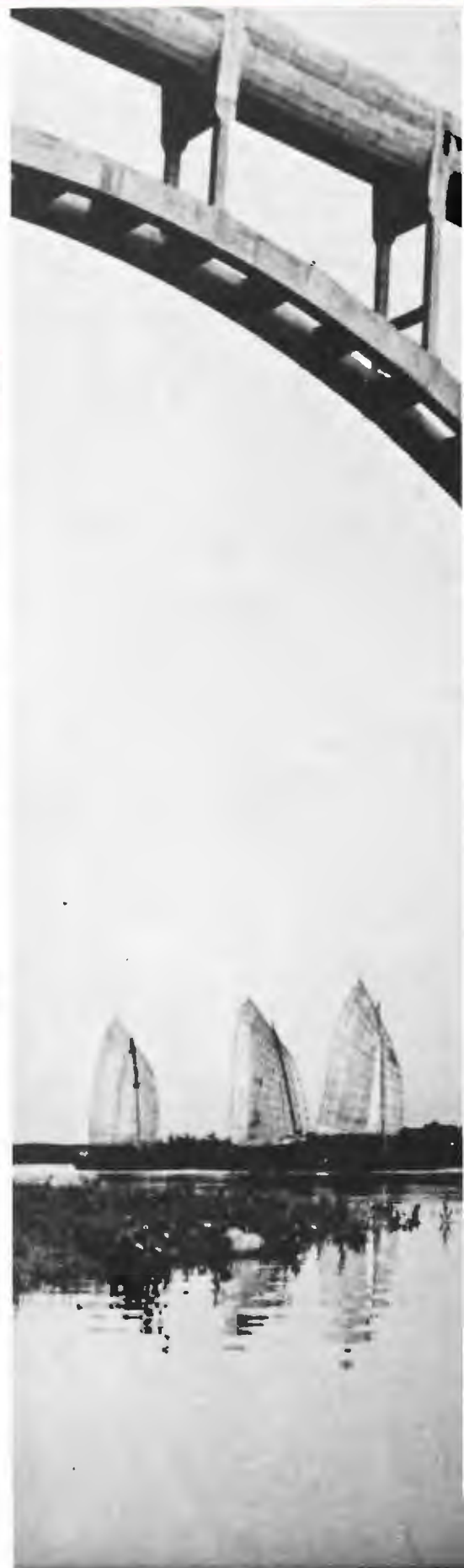
An aqueduct in a Chinese countryside.
