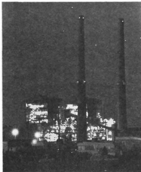
A Montana Power and Light Co. power plant at Colstrip, Mont., is lit up like a Christmas tree at night.
