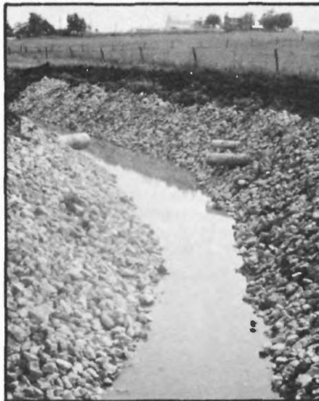
Rocks have been placed along the banks of this stream to reduce erosion and washing of mud into the Black Creek watershed.
